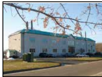
Research Drive Lab / Office
