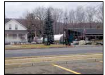
Amity Road Development Site
